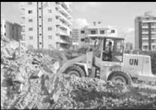
Clearing debris from Israeli bombardment of apartment building in Tyre July 2006
